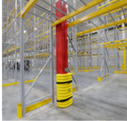
Building Column Guards
