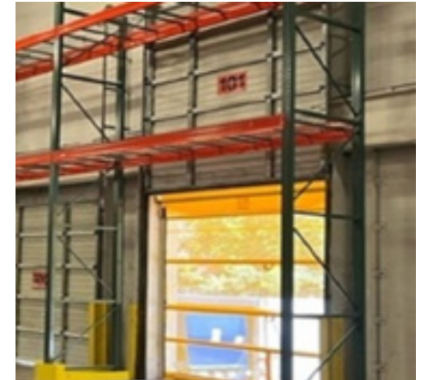
Over Dock Racking
